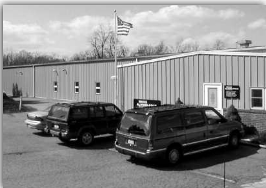
▲ 30,000 sq. ft. production facility in Elizabethtown, Pa.
